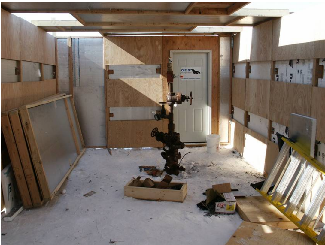
Figure 7 – Umiat #8 wellhead inside wooden enclosure
